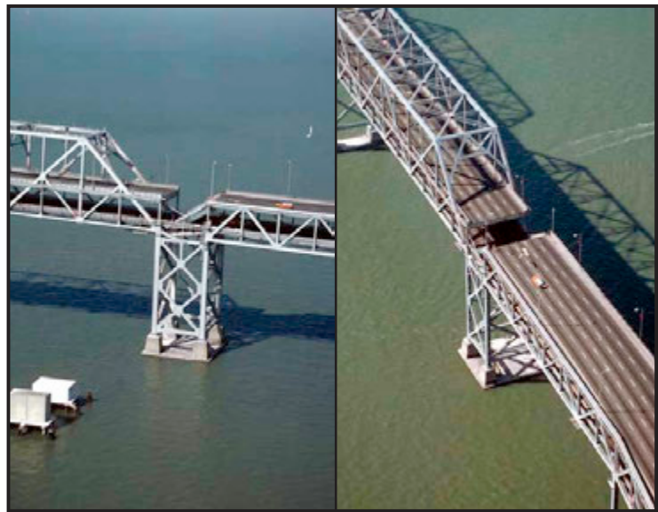
Figure 1.1. Two aerial views of the collapsed section of the San Francisco–Oakland Bay Bridge. (Photo: C.E. Meyer, USGS)
