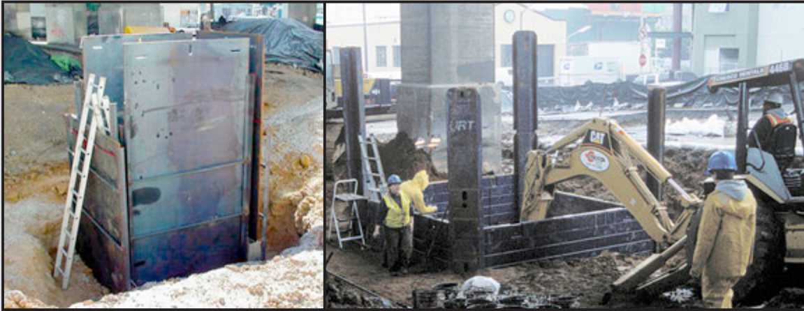
Shoring for Well 6, Block 9. After several months' delay this custom shoring (shown on left, as installed), designed by the construction contractors was deemed too dangerous and ineffective to use. It was replaced with this commercial version (on right). (Photo on left, courtesy of Dani Renan)
