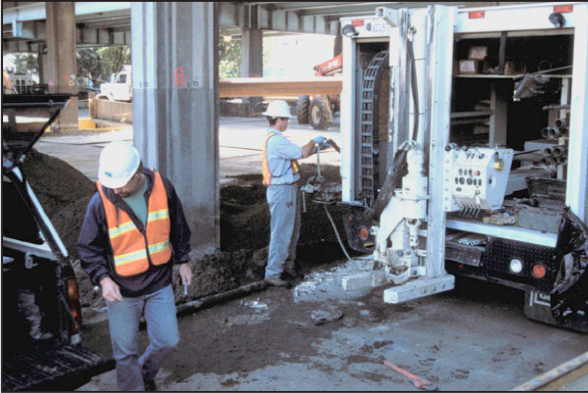
Geoprobe setting up to drill cores at Bent L72 on Block 3 of the SF-80 Bayshore Seismic Retrofit Project.
