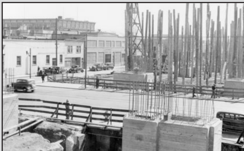
This 1935 construction photograph from Block 9 across Third Street shows bent footings in place and false work piles being driven on Block 10. (Photo courtesy of Bay Bridge Archive, Caltrans District 4, F15-206)
