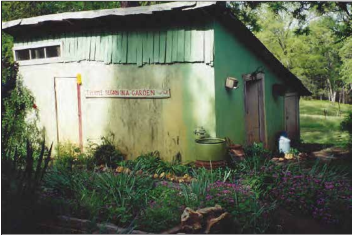
Figure 1. A shed-roofed utility building with plywood walls and iron-sheet roofing, the outbuilding was likely constructed by Dick and Helen Hoffman between ca. 1965 and 1990 (Photo courtesy Joanne Thompson).
