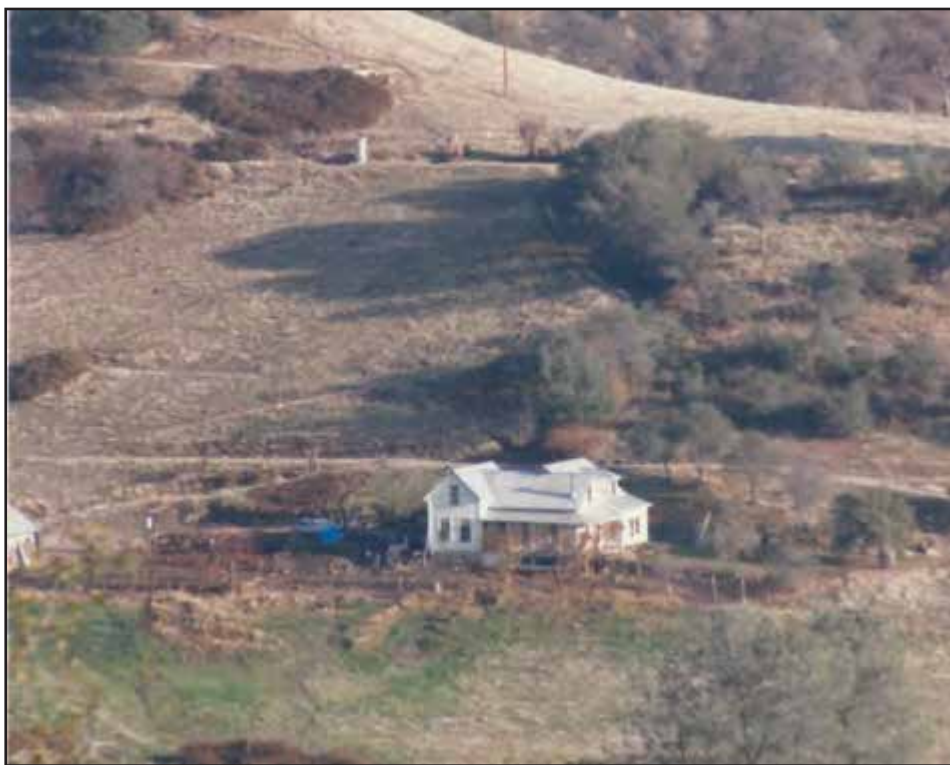
Figure 1. Curnow ranch house in 1986, view to east, showing the three stages of construction: the N-S running portion with porches (ca. 1870); the narrow E-W addition on the northeast corner (ca. 1902), and the rear eastern N-S addition of ca. 1920s. (Photo courtesy Julia Costello).
