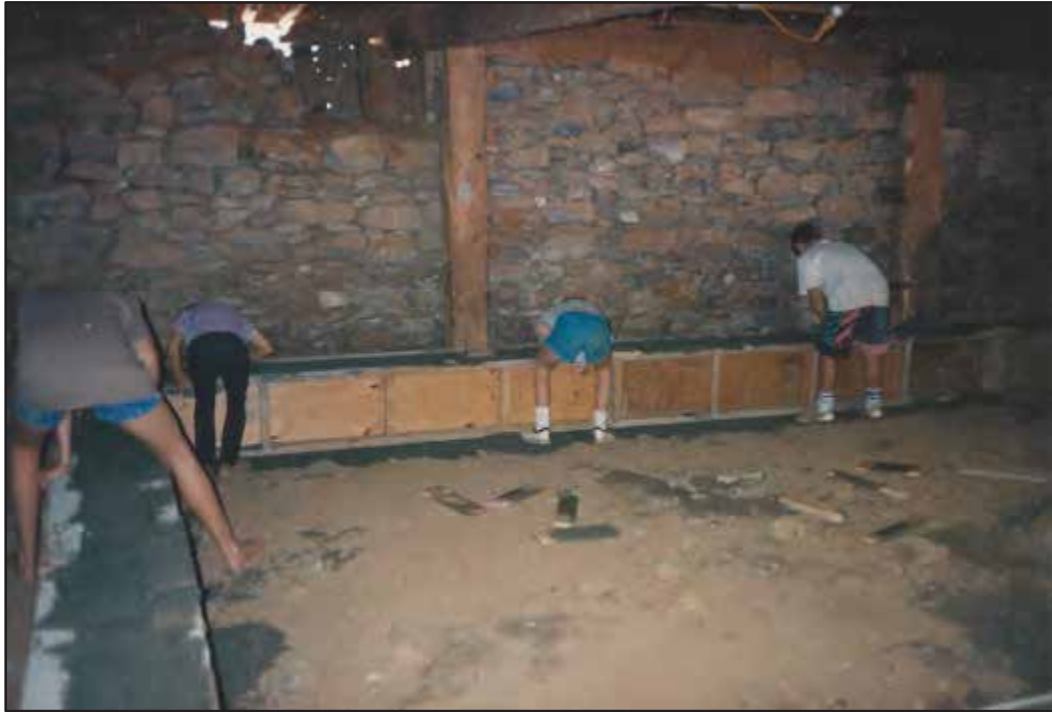
Figure 5. The interior of the south wall of the basement (Ctx. 300) has been rebuilt and a concrete sill foundation is being poured in the frames; September 1987. (Photo courtesy Linda Mariani)
