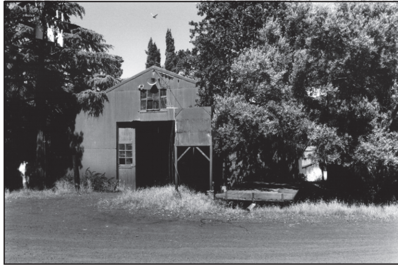
Oscar Starr's Machine Shop. Starr built and used this steel-frame shop to experiment with Caterpillar-tractor technology. Clad with corrugated-iron sheets on the wall and roof, it must have gotten rather warm in the summer and noisy during the wet winter months. (Courtesy Dell Upton.)
