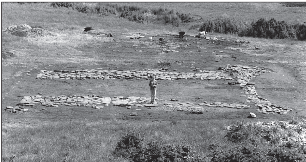
Barn Stone Floor. This is what remains of the large barn that once stood at the Weymouth/Rose site on the east side of the Kellogg Creek Valley. The stonework is extensive and forms both foundation and partial floor. There is no mortar between the stones, but they are carefully laid in an interlacing network that keeps the structure strong.
