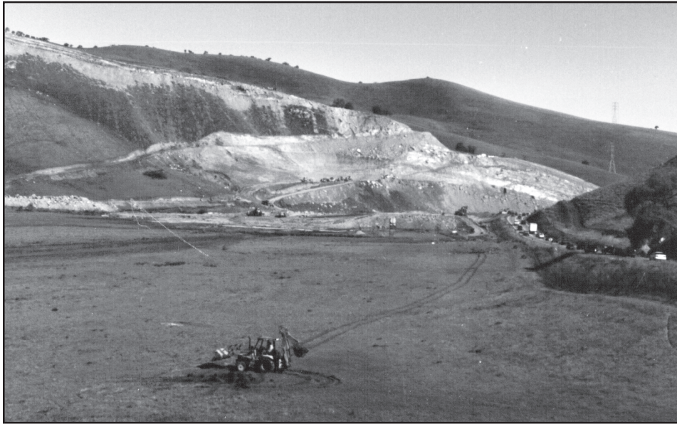
Construction of Los Vaqueros Dam, 1996. The hills at the north end of the valley are graded while soil is mined from the valley floor to construct the 192-foot dam that will hold back the waters of the new reservoir. ( Photograph courtesy Jack Meyer. )
